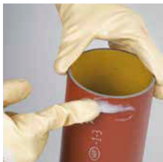
Apply a small amount of jointing lubricant on the pipe or fitting spigot, rather than on the rubber gasket to ease the fixing.
