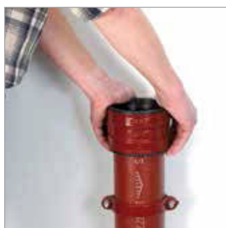
Push joint over the end of pipe, ensuring the central register is abutted against the spigot edge evenly.
