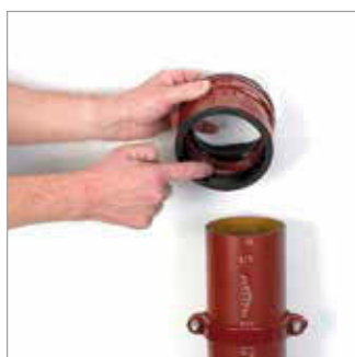
Apply a small amount of jointing lubricant on the lip of the rubber gaskets, both ends to ease insertion of pipe/fittings.
