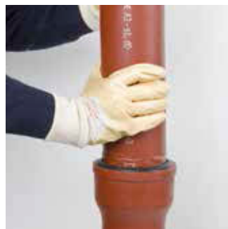
Push joint into the pipe or fitting socket, ensuring the central register is abutted against the spigot edge evenly.
