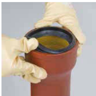
Insert the gasket into the socket
