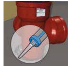
Seal the openings with cement or sealant.
