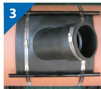
**3.** Bars must be centered and positioned overlapping the initial set of clamps.
