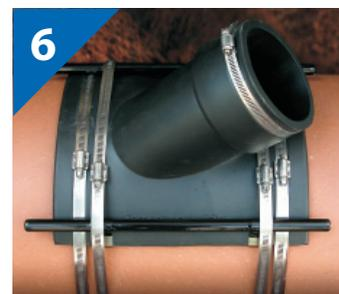
**6.** Test for leaks prior to backfilling
