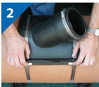
**2.** Attach the reinforcing bars to the boss junction by sliding the clips under the boss junction.
