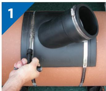
**1.** Install the appropriate Fernco Flexible Boss Junction as needed. Tighten clamps to 60 inch-lbs. torque.
