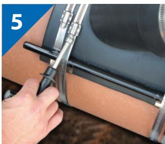
**5.** Tighten clamps to 60 inch-lbs. torque.
