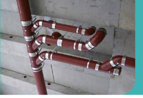
all normal maintenance processes, including high-pressure jetting, without being damaged. They have undergone a high-pressure test according to Swiss standard SN 592 012.
