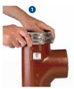
Push the supplied assembled coupling onto the pipe spigot so that it abuts on the central register of the elastomer gasket.
