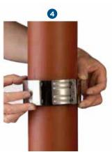
Place the steel strap around the sealing gasket.
