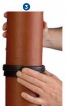
Install the next spigot and unfold the gasket half back.
