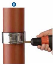
For PAM CV-CE couplings: Alternately tighten the two tightening screws uniformly and hand tight. The threaded plates must come together parallel to avoid any deformation.
