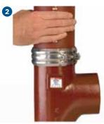
Push the next pipe spigot into the other end of the coupling.
