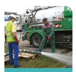
The S and Plus ranges, assembled and anchored, have successfully passed a high-pressure jetting test: cleaning pressure of 120 bar from the pump, which means 100 bar at the nozzle outlet, without leaks or misalignment.
