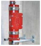
We recommend positioning the first stack support pipe at the base of the first floor, and then every subsequent fifth floor, in the case of a standard average 2.5 m between floors, or more generally every 15 m.
