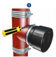
1.Insert the PAM KONFIX rubber connector loosely onto the pipe until the stop point is reached. Then secure to the pipe by tightening the hose clamp screw.
