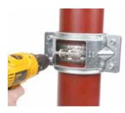
Tighten the screws crosswise alternately so that the two plates are put in parallel with the same spacing.
