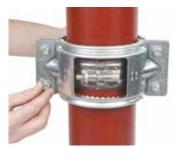
Insert the four screws to fix the two parts together loosely.
