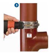
Tighten the screw to "zero gap" position, i.e. fully closed, with a ratchet spanner or electric screwdriver.
