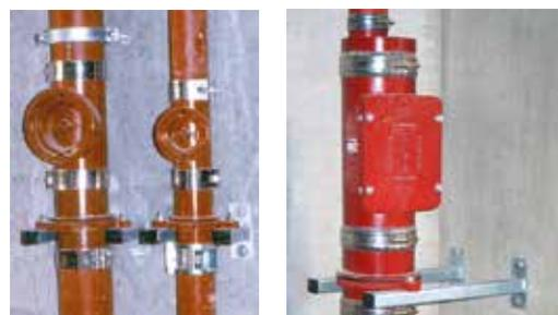
We recommend positioning the first stack support pipe at the base of the first floor, and then every subsequent fifth floor, in the case of a standard average 2.5 m between floors, or more generally every 15 m.
