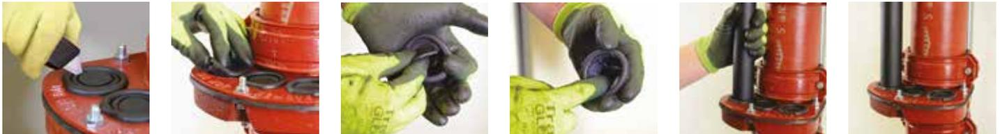
1. Cut the appropriate groove for 32 mm or 38 mm waste connections (100 mm manifold only), remove the grommet and tear out the centre disk where required.
