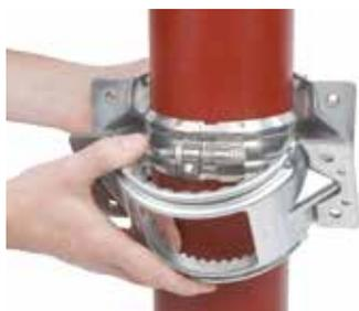
Position the two half parts of the PAM grip collar uniformly so it encircles the pipe in parallel. The grip collars must be positioned so that the apertures fit over the coupling's fixing bolts and the teeth are directly located onto the pipe.
