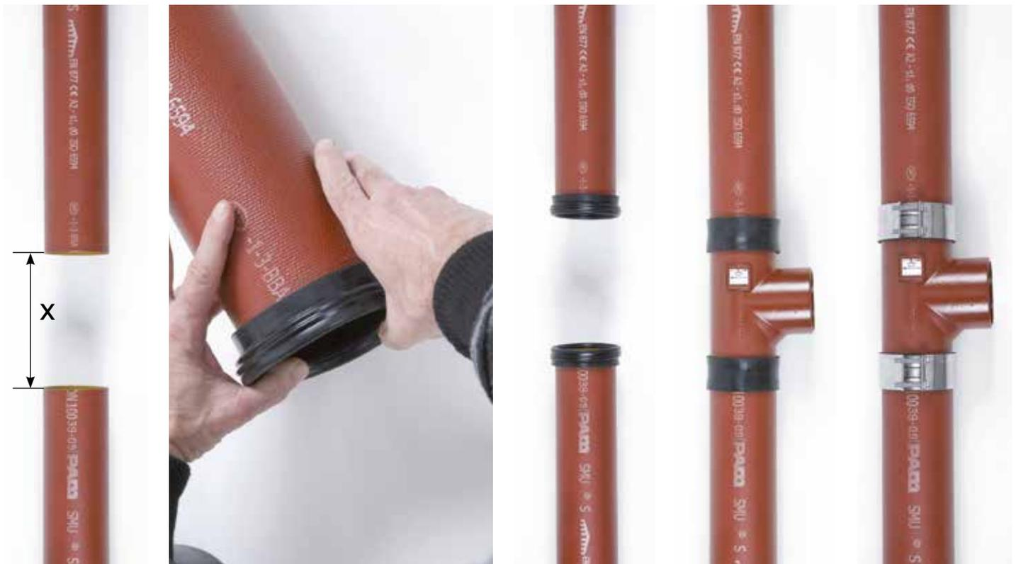
$X = \text{fitting} + 15 \text{ mm}$
