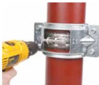
Tighten the screws crosswise alternately so that the two plates are put in parallel with the same spacing.
