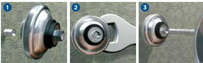
1. Fasten the PAM Acoustic Dampener to the thread in the wall with an open-end wrench.
