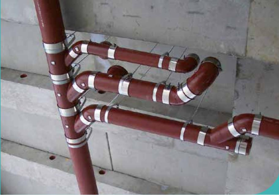
all normal maintenance processes, including high-pressure jetting, without being damaged. They have undergone a high-pressure test according to Swiss standard SN 592 012.
