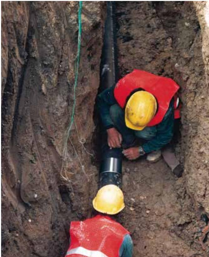
Buried systems are subjected to ground loadings which can cause shearing strain on couplings. **For these applications, it is therefore recommended to use wider couplings, and to use the “all stainless steel version” of the steel couplings** to avoid corrosion due to the aggressiveness of the ground.
